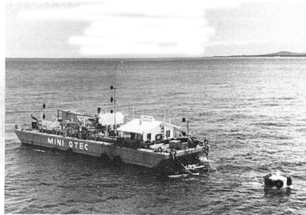
Fig. 3 Mini-OTEC moored off Keahole Point in Hawaii
